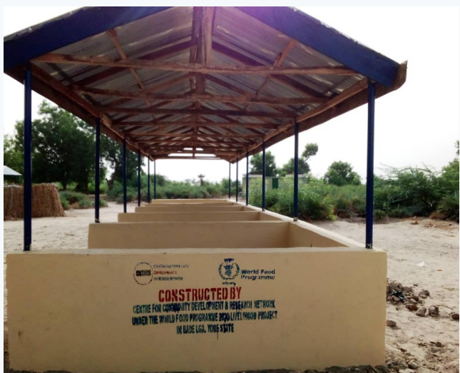
A newly Constructed Market Shed under the WFP livelihood Project in Bade
