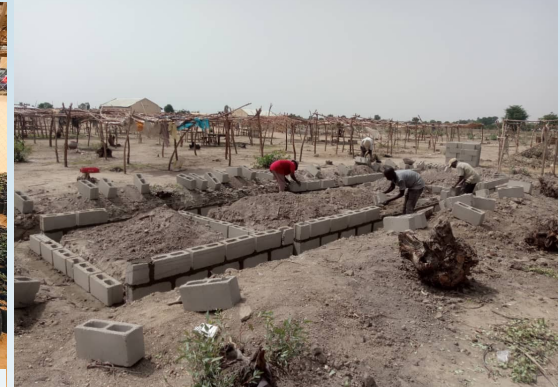
Ongoing construction of Market shed in Madagali
